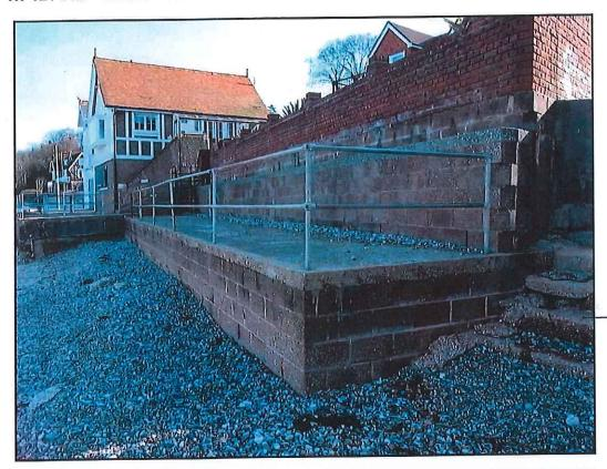
NOTES: Concrete step block. Steel railing.
