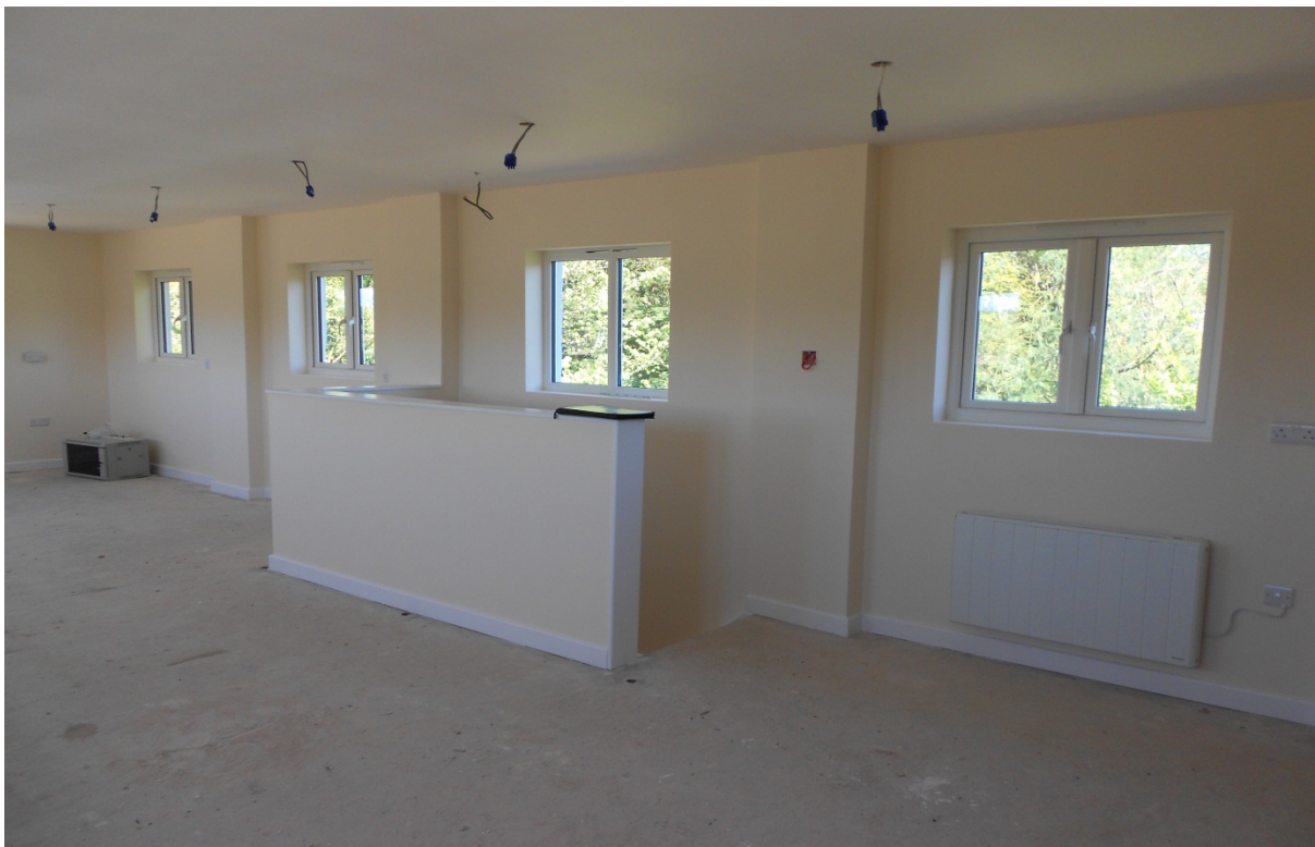
FIRST FLOOR OF PREMISES SHOWING WINDOWS FACING RESIDENTIAL PROPERTIES
